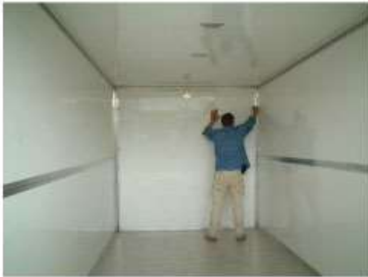
Erecting the end panel
