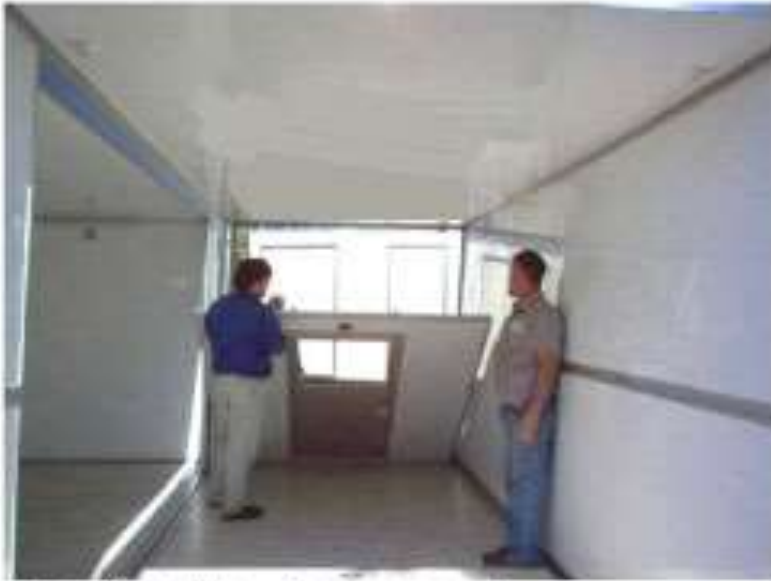
Erecting the door panel
